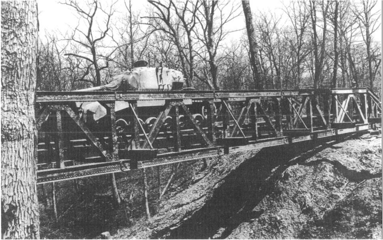
Figure 2-8. T6 aluminum fixed bridge.
