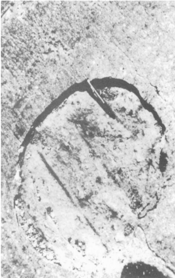
Figure 5-8. Large spall.
