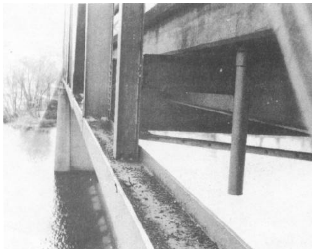
Figure 8-23. Lower chord of a riveted truss.
