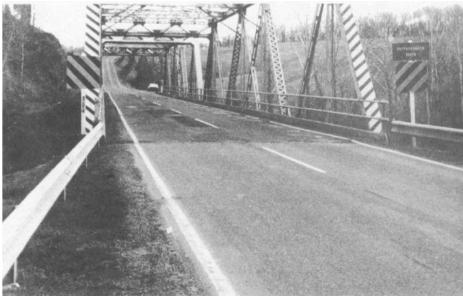
Figure 8-35. Appropriate markings for clearances on civilian bridges.
